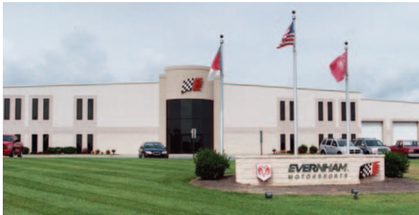
Evernham Motorsports' Statesville, N.C. complex has three facilities for engineering, administration, fabrication and R&D as well as an adjacent airstrip for their three corporate airplanes.
